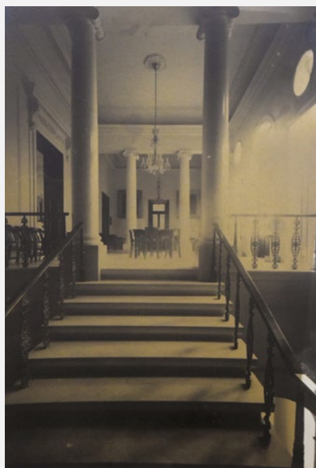
Part of a series of old photos of the Chamber's interior spaces.
