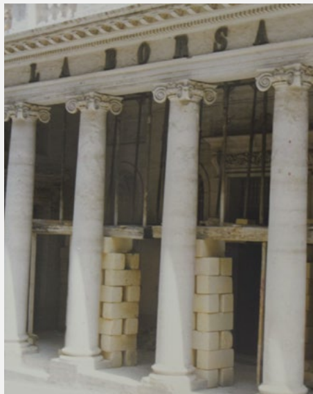
Renovations on the Chamber's portico.
